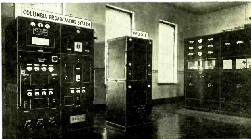
Close-up of the transmitter panels of W2XE, "CBS" high frequency station.
