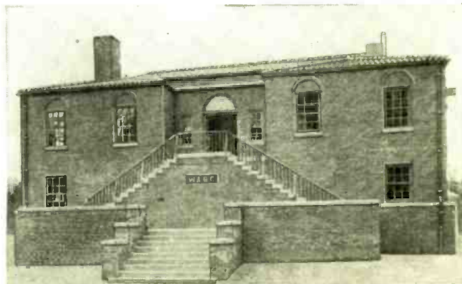
The transmitting equipment of W2XE is housed in this building at Wayne, N. J., about 25 miles from New York.
